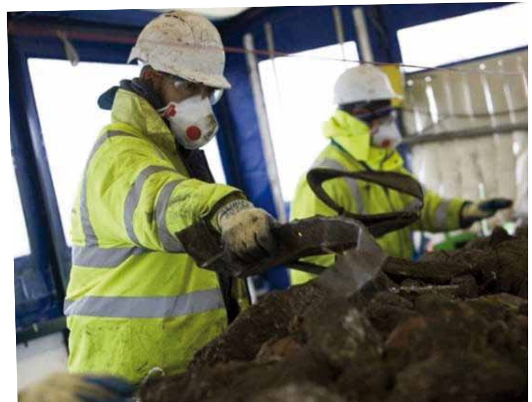
98 per cent of demolition waste was reused or recycled.
