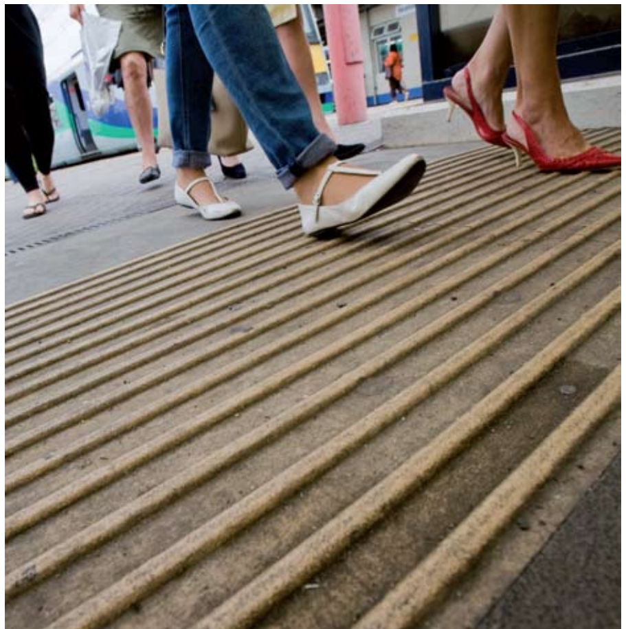
Tactile warning surfaces on platforms and staircases will help to make stations more accessible to people with visual impairments
